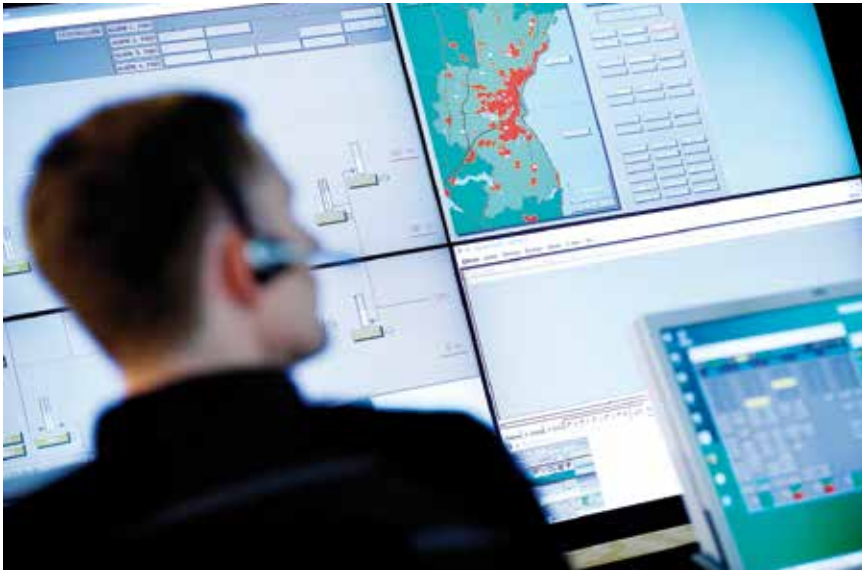
CONTROL CENTRE IN AARHUS – PHOTO BY OLE HARTMANN SCHMIDT
