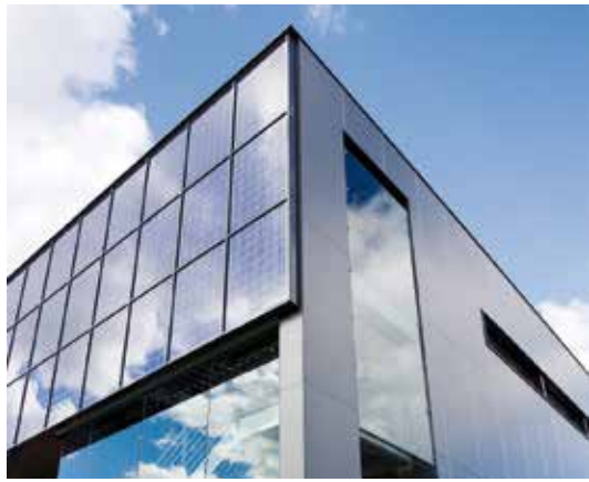
SOLAR PANELS AT WATERWORKS – PHOTO BY VCS DENMARK
