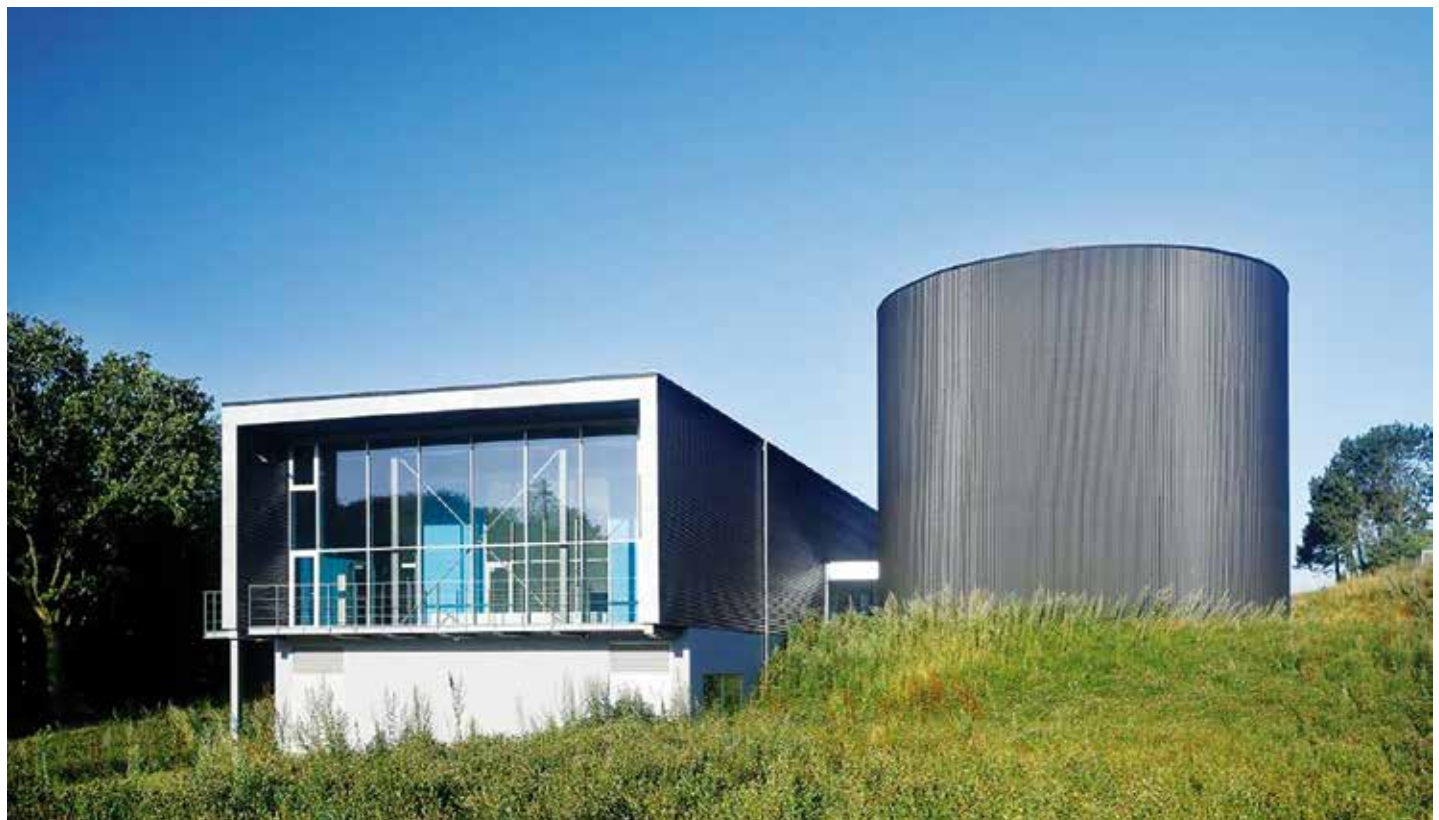
TRUELSBJERG WATERWORKS IN AARHUS – PHOTO BY OLE HARTMANN SCHMIDT
