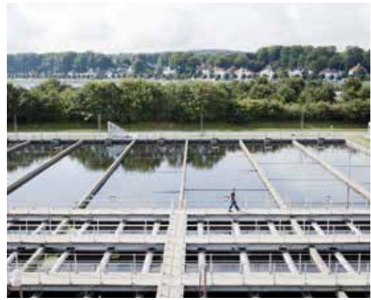
MARSELISBORG WASTEWATER TREATMENT PLANT IN AARHUS – PHOTO BY AARHUS VAND
